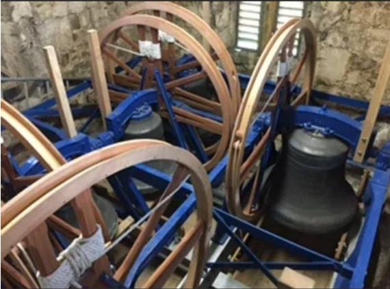
With a steel frame, the set is hung in a balanced way so as to not impose excessive forces on the tower structure when the bells are being rung. The vertical and lateral forces are up to 4 and 2 times the bell's weight, transmitted to the tower
